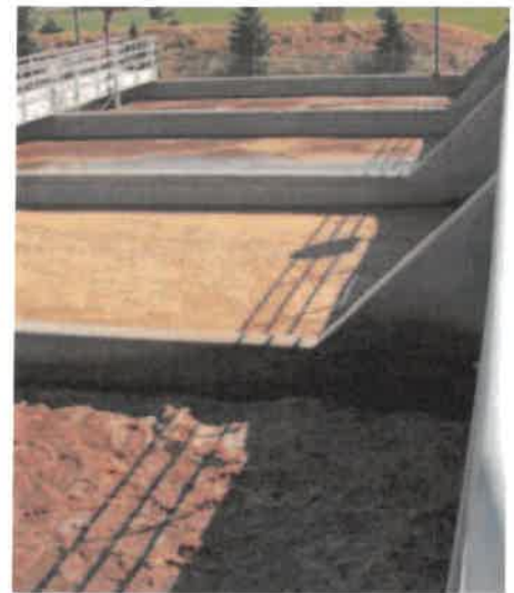
Biological Oxidation treatment at Medical Lake Water Reclamation Facility.
